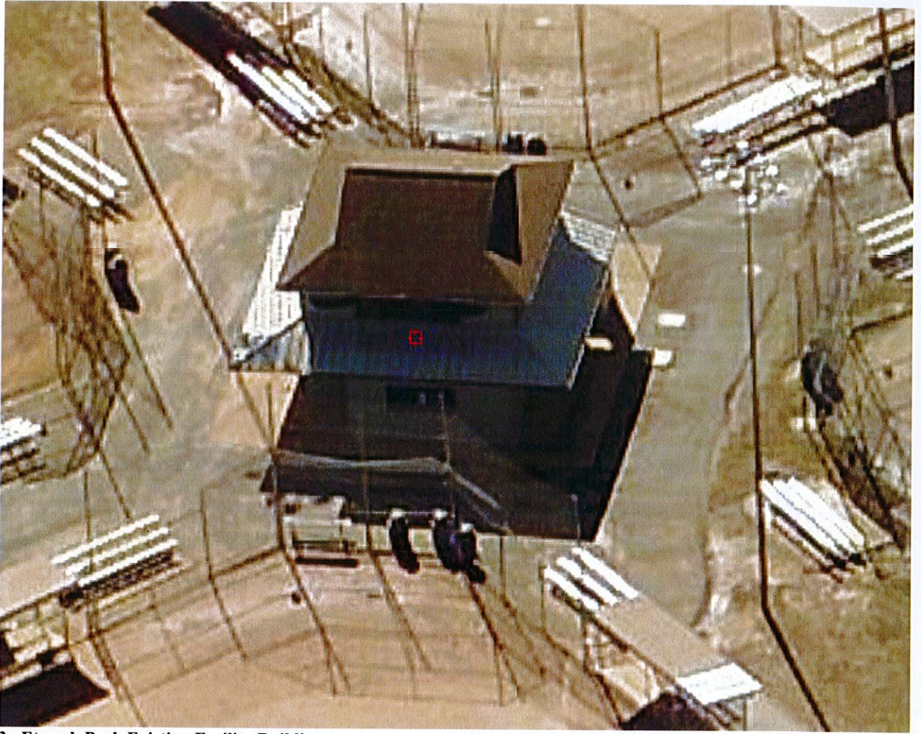
3. Etowah Park Existing Facility Building
