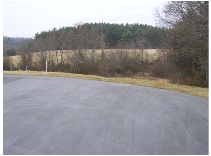
2. View of the end of Waters Edge Drive looking west.
