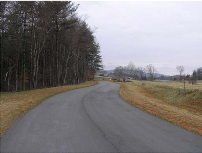
3. View of the center of the project site on Waters Edge Drive looking north.
