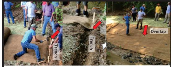
Matting 1) Lay start of matting in trench and tamp in 2' oak stakes with nail on end. Add every 1.5' to top of trench. Overlap extra matting rolls by 1'.
