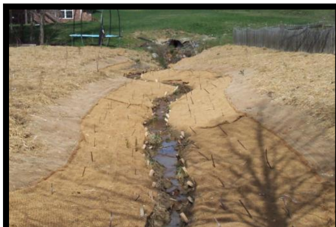
Matting 4) Once all the matting is laid out and secured with stakes, cover trenches with a few inches of soil, tamp it down and lightly cover top edge with straw to undisturbed landscape.
