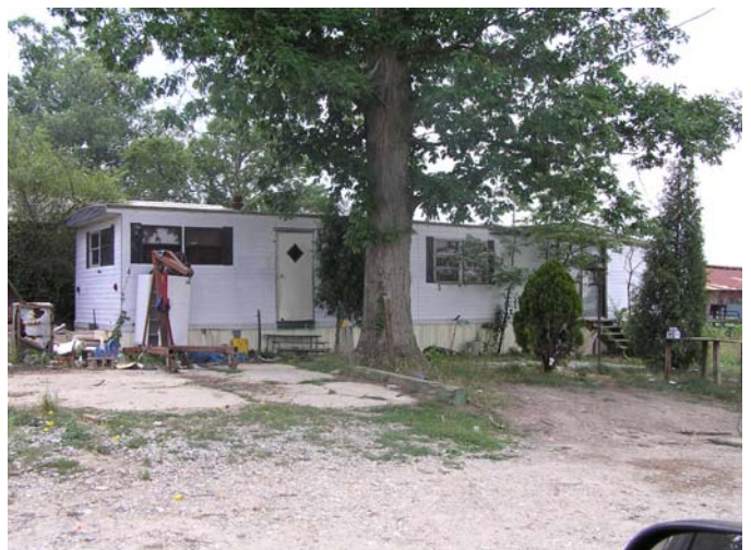
4. View of the existing Residential Structure D on Tract 1, looking west from Tap Root Lane.
