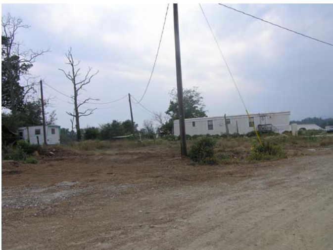
5. View of the existing Residential Structures E and F on Tract 1, looking west from Tap Root Lane.
