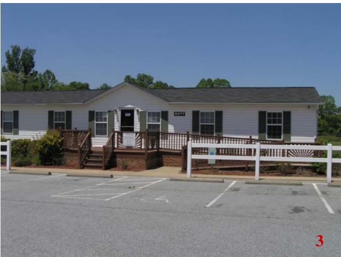
3. Existing business (modular home sales) on remainder tract along Hendersonville Road (Highway 25N)
