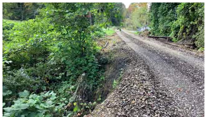
Steep slopes adjacent to the existing railbed
