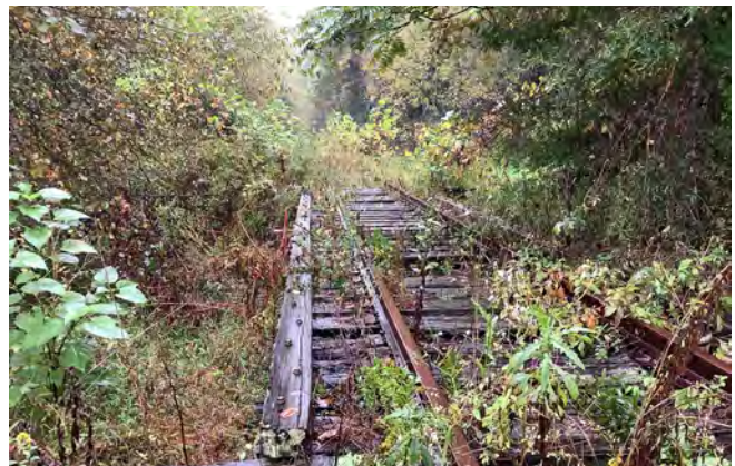
The existing railroad bridge along project corridor
