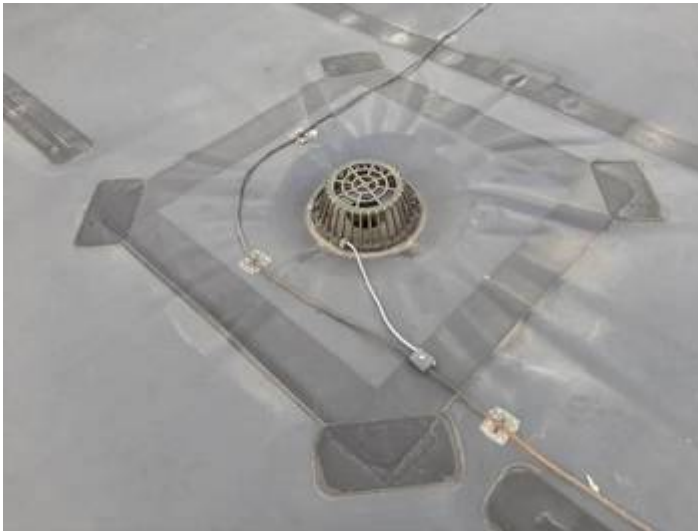
Figure 2 – Roof at roof drain
