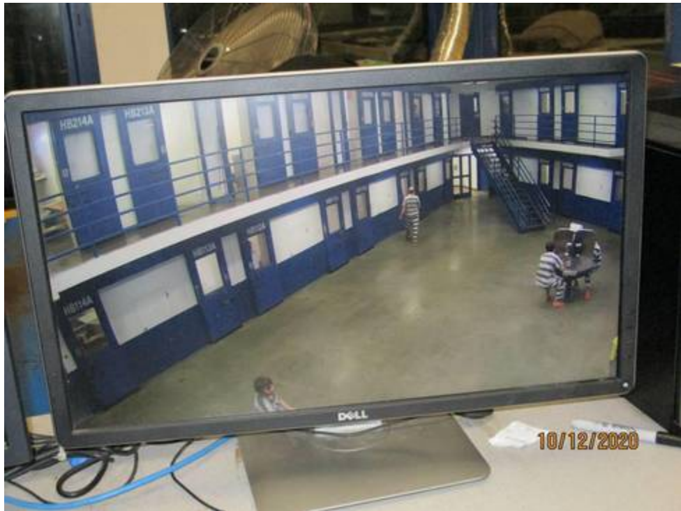
Figure 23— IP-CCTV Spot Monitor at control stations (typical)
