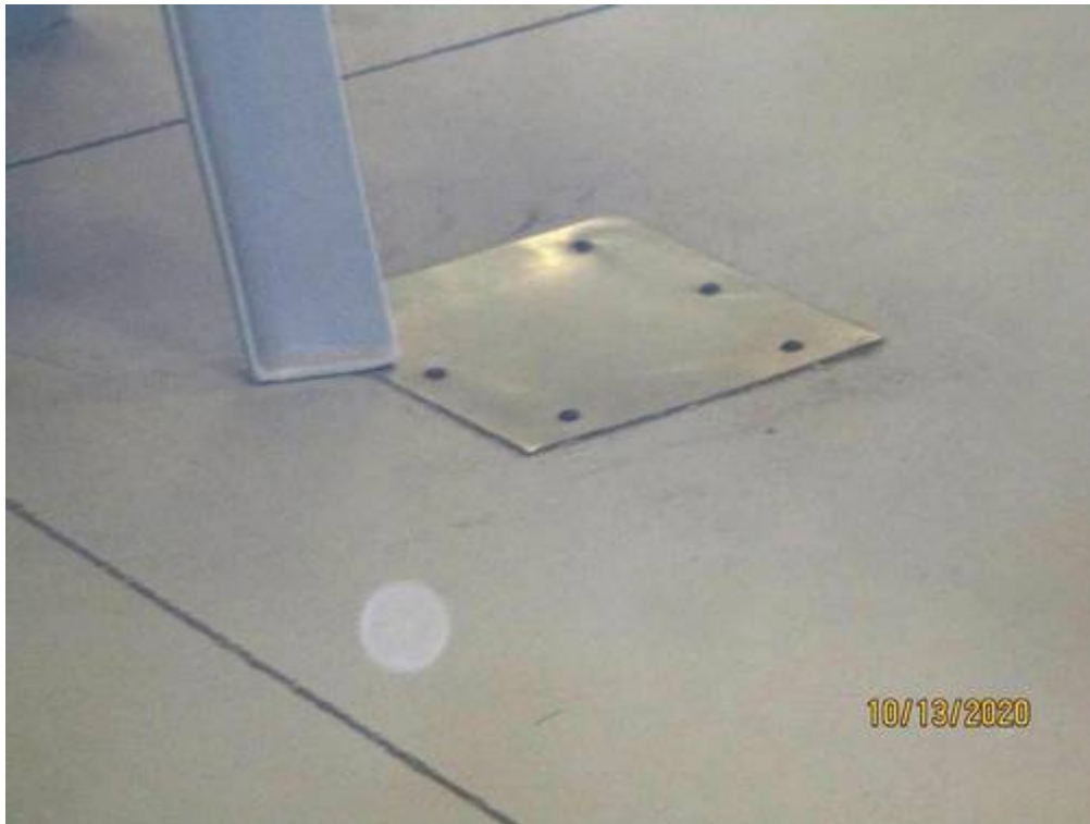
Figure 24— Male Housing Unit C future Direct Supervision control box (typical also of D Unit)
