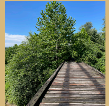
Rail bridge over the French Broad River.
