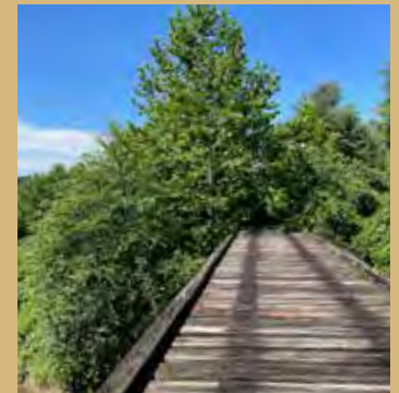
Rail bridge over the French Broad River.
