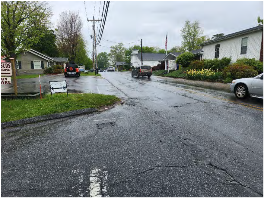
Street view of White St from the subject property facing W
