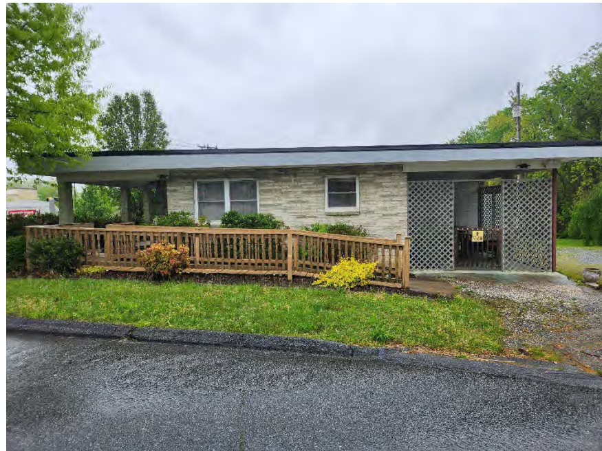
West side of subject's improvements
