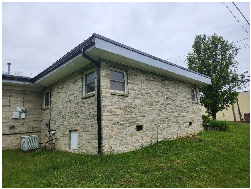
East side of subject's improvements
