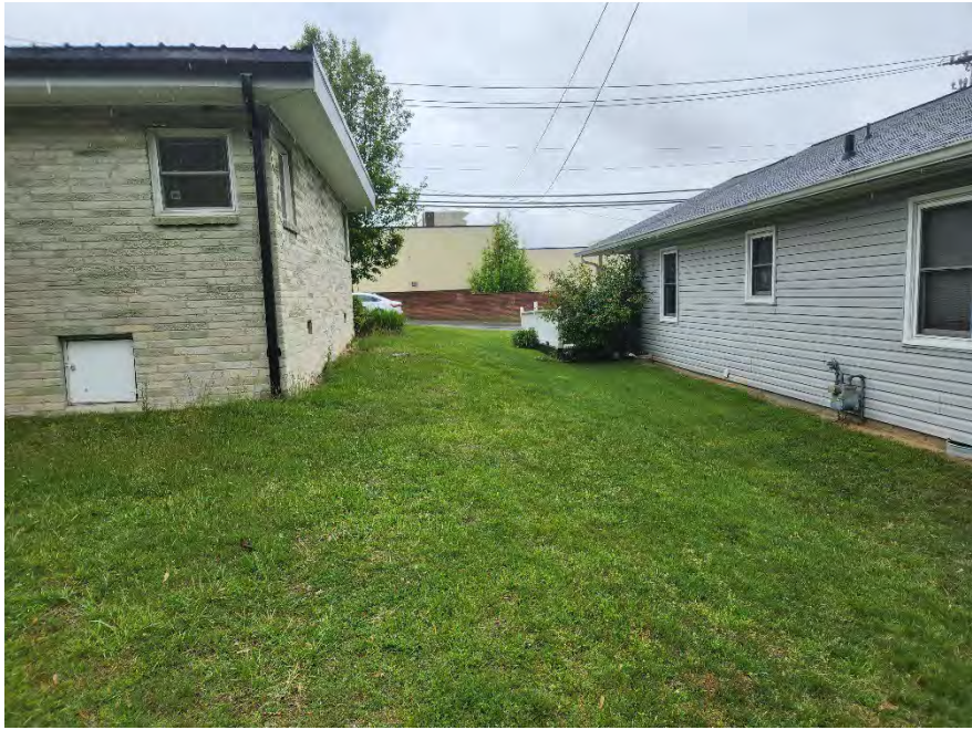
East side of subject's improvements
