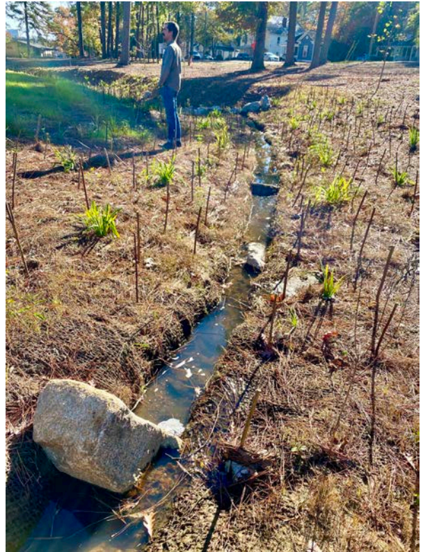
Cover image: Portion of the daylighted stream after construction showcasing the newly planted live stakes.
