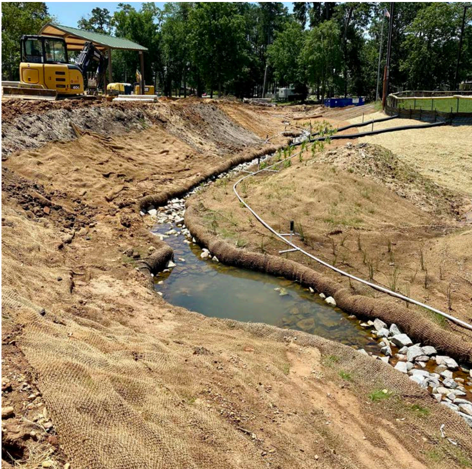
Cover image: Portion of the daylighted stream after construction showcasing the newly planted live stakes.
