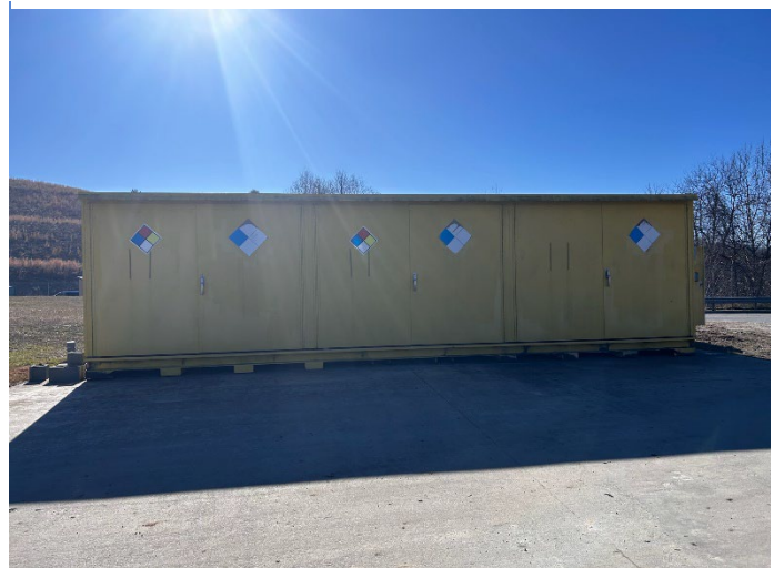
Photo 1: Current HHW building at the Convenience Center
