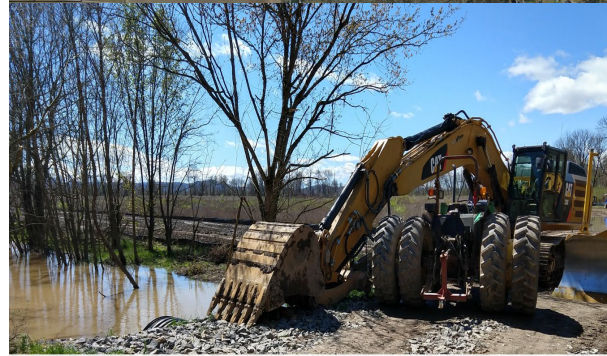
Restoration: Grading and Construction
