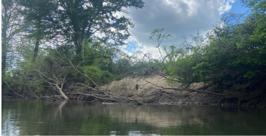
French Broad River Bank Erosion
