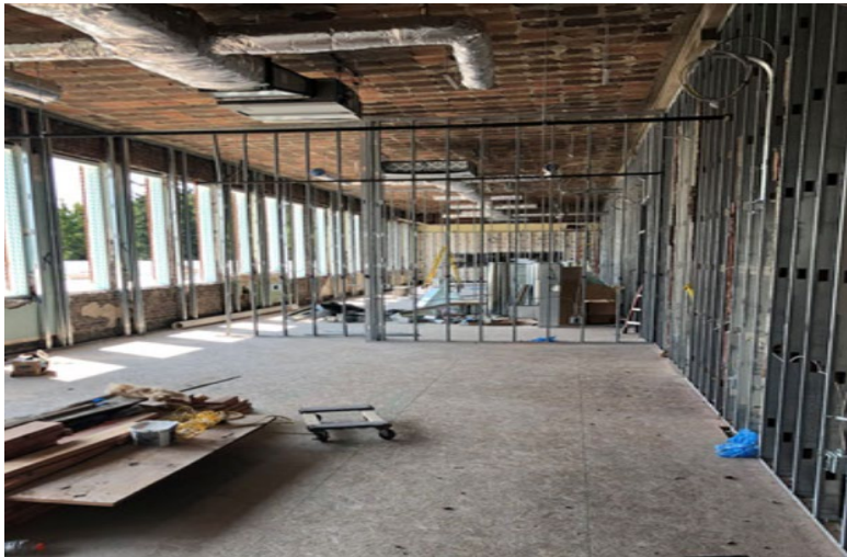
Interior of Stillwell Building at Hendersonville High School.
