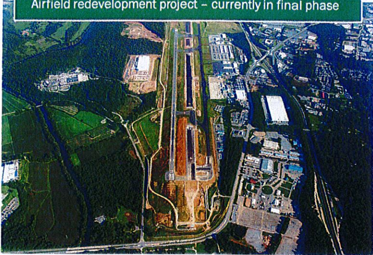
Airfield redevelopment project – currently in final phase
