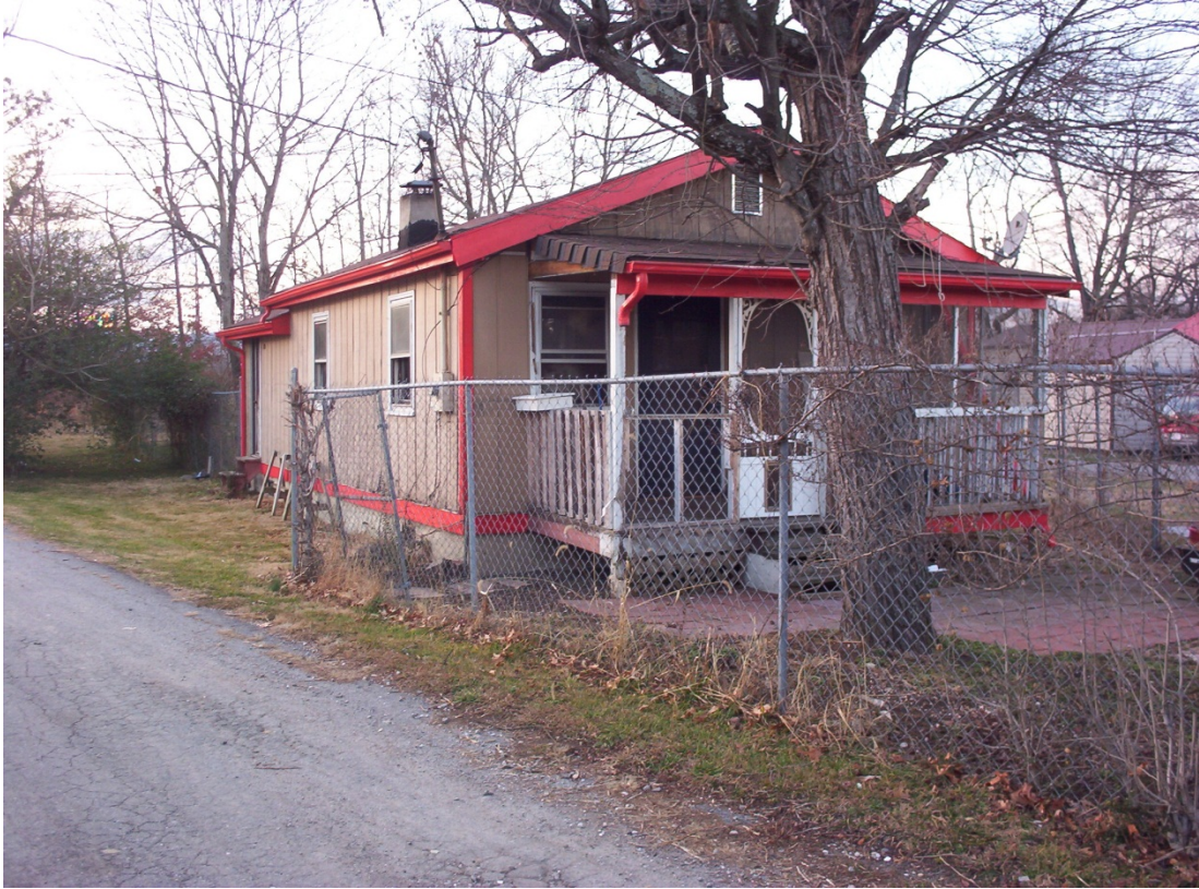
Looking West Front of Building
