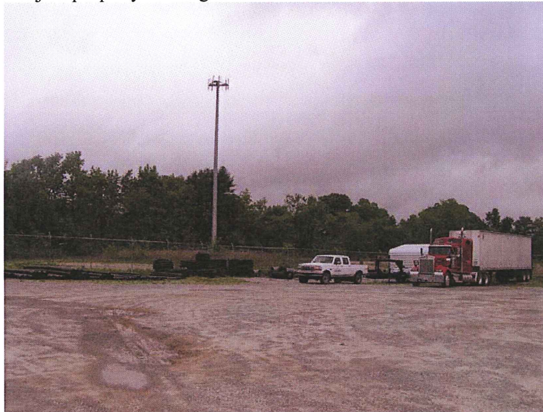
Subject property looking northeast at cell tower
