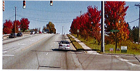
Spartanburg Hwy & Glover Street – Existing Signage Location #2 on approach, traveling east.
