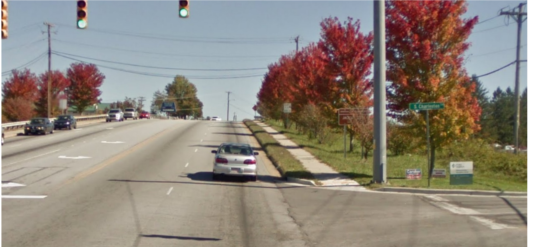
Spartanburg Hgwy & Glover Street – Existing Signage Location #2 on approach, traveling east.
