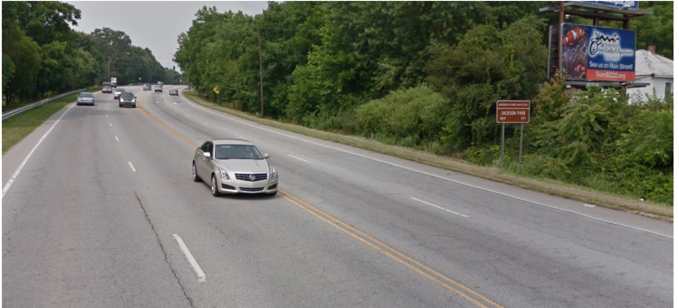
Four Seasons & Ashe Street – Existing Signage Location #1 on approach, traveling west.
