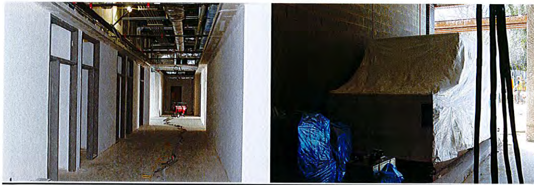
Air handling unit
