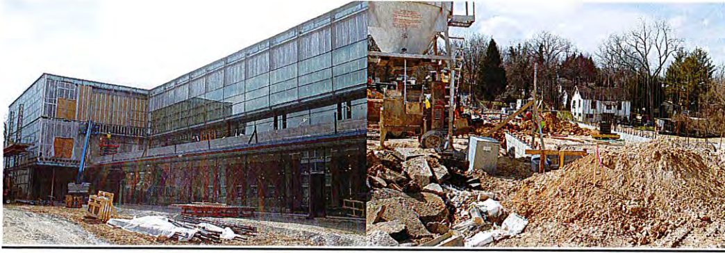
Glass installation should be complete in April.
