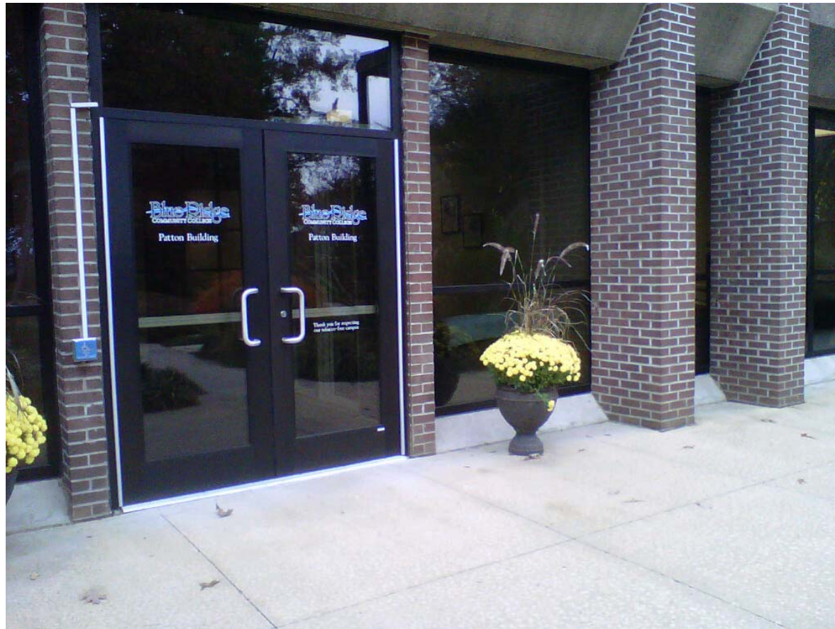
Example of New Doors for Patton and Con Ed
