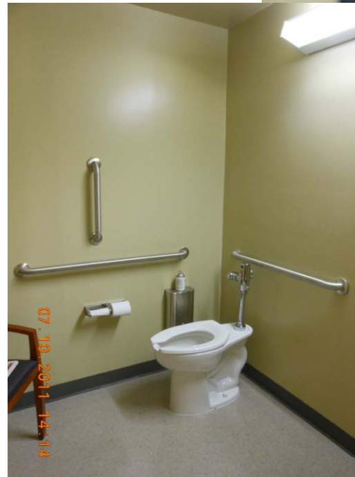
Patton Restroom Renovation
