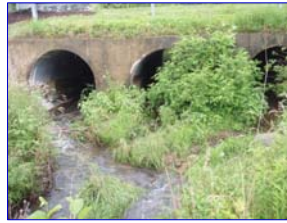
Rugby Middle School Culvert
