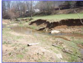
Severe Bank Erosion along Reedypatch Creek
