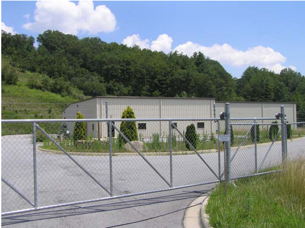
View of structure on Tract 1 looking east from Old Hendersonville Rd
