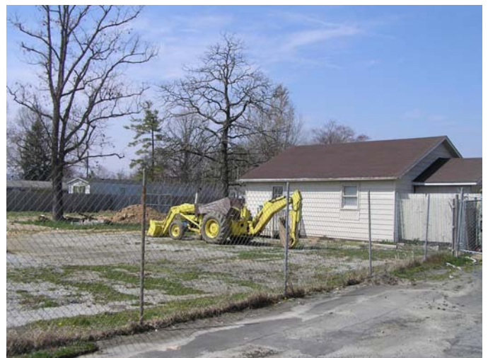
12. View of commercial use on Dairy Rd looking north.
