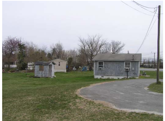
10. View of Subject Area west of Hendersonville Rd (US Hwy 25N).
