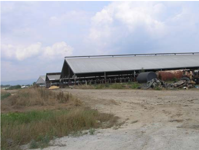
11. View of existing structures for agricultural/industrial use on Tract 1, looking east from the Tap Root Dairy Road.
