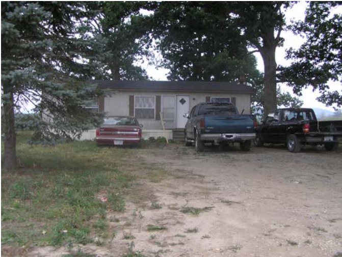
15. View of the existing Residential Structure I on Tract 2, looking west from Tap Root Dairy Lane.
