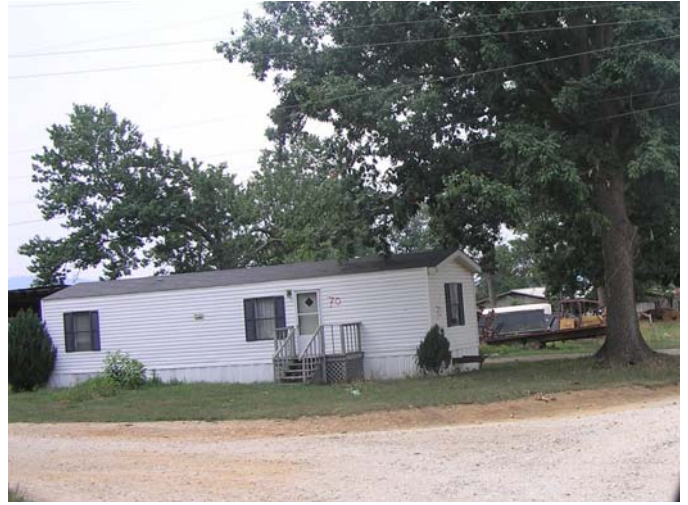
2. View of the existing Residential Structure B on Tract 1, looking west from Tap Root Lane.
