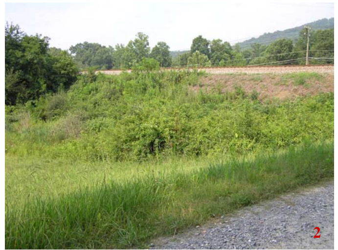
2. View of Norfolk Southern Railway, which runs between Asheville Highway (US 25 N) and the Subject Area, looking east from Teresa Lane.
