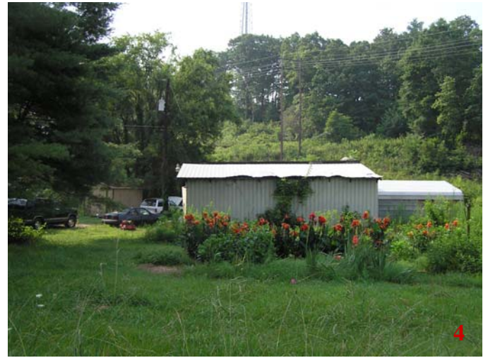
4. View of three (3) existing residential accessory structures, looking southeast from Teresa Lane.
