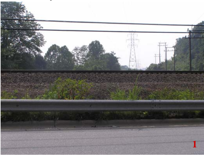
1. View of Norfolk Southern Railway, which runs between Asheville Highway (US 25 N) and the Subject Area, looking west from Asheville Highway.
