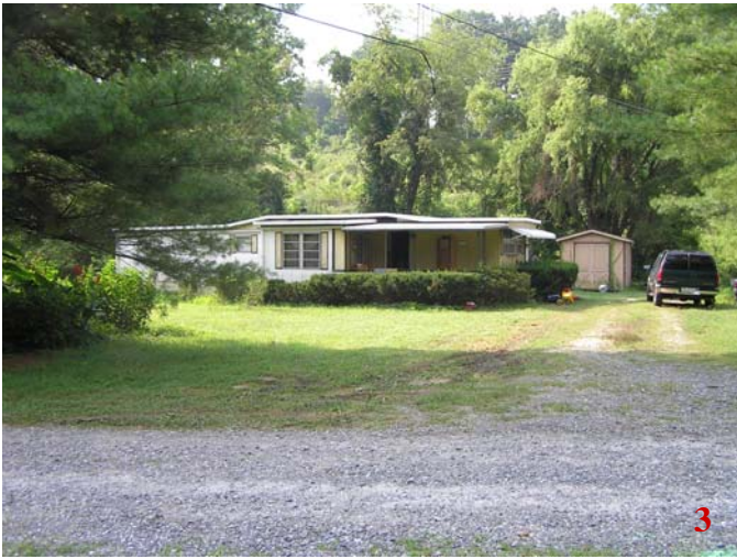
3. View of existing structures (manufactured home and storage building) and point of access to the Subject Area property, looking south from Teresa Lane.
