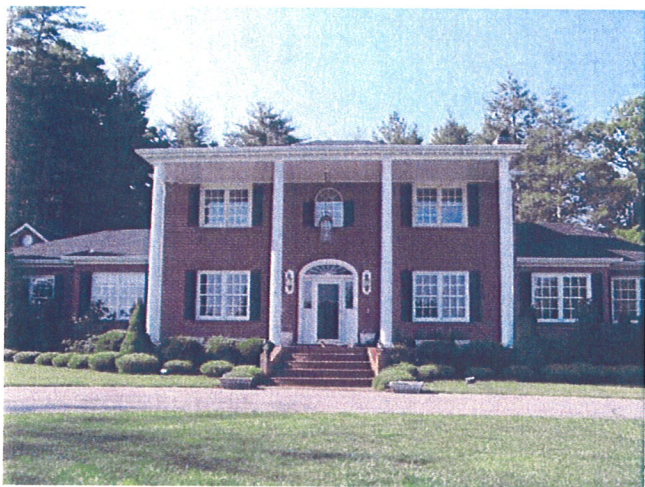
View of existing residential structure looking south.
