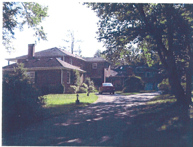
View of existing residential structure looking east along the private drive.
