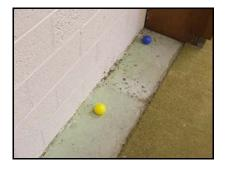
Exterior walls are 12-inch cavity brick walls. Partition walls are brick walls. There was some cracking in the interior masonry wall where it intersects with the exterior wall. It is assumed that most of this cracking is caused by either thermal movement of the building or soil settlement under the wall. Additional detailed investigation is required to find the definite cause of the cracking in the wall. All the remaining walls appear to be in good condition.
