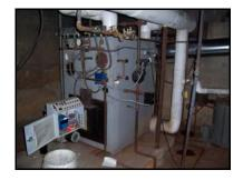
The existing heating for the main School building consists of a basement oil-fired steam boiler and steam radiators installed throughout the building in various locations. The boiler has 892,000 BTUH steam output, appears in good working condition, and could probably be re-used in the building's new life. The boiler level control appears to have had a manual reset button installed and should be adequate. All building steam radiators, controller, and steam traps could be re-used if the occupants
