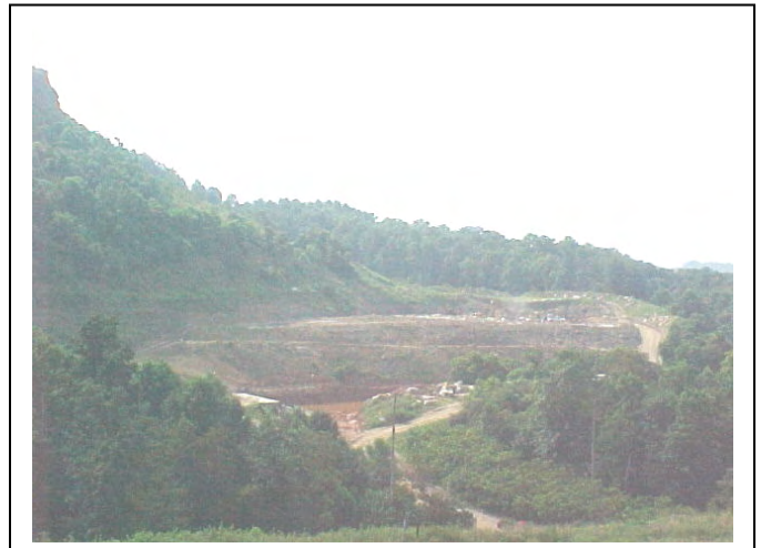
View of the Henderson County Landfill.
