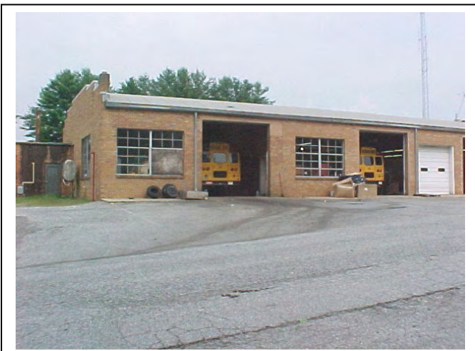
Henderson County Public Schools bus maintenance garage.
