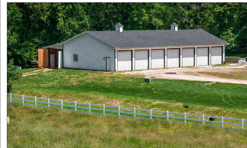
EXISTING BARN/FUTURE SPA-WELLNESS CENTER
